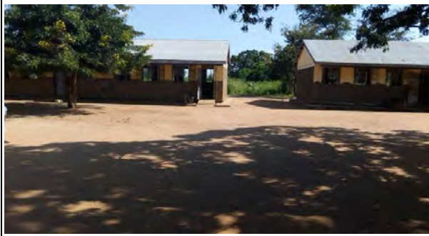
Classroom / Administrative Block
