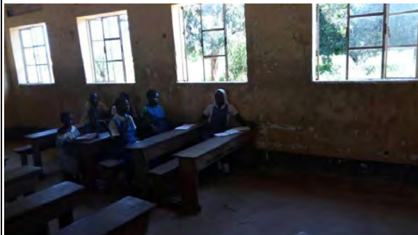
Classroom / Administrative Block (Interior)
