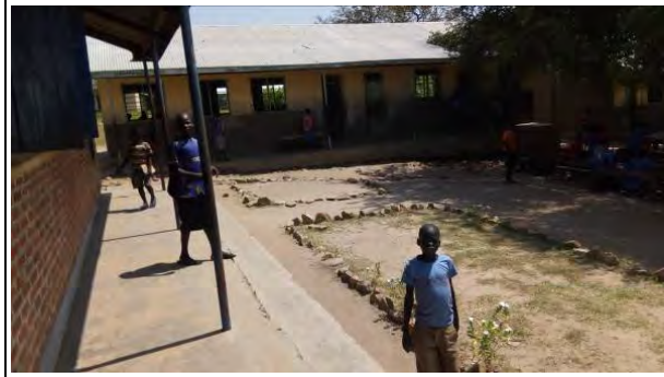
Classroom / Administrative Block
