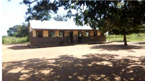
Classroom / Administrative Block
