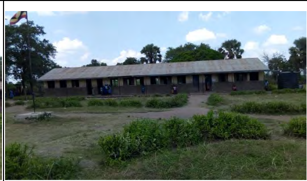
Classroom / Administrative Block
