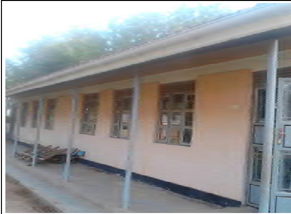
Classroom / Administrative Block
