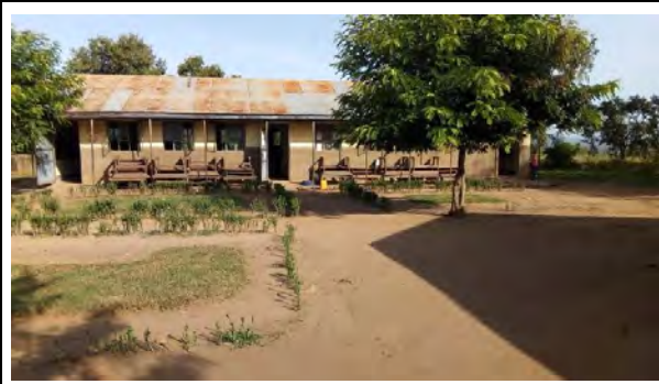
Classroom / Administrative Block
