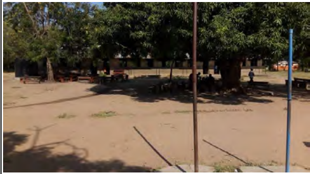
Classroom / Administrative Block
