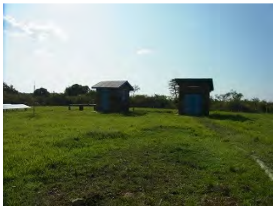
Distant view of Itula Water System's pump room. (Itula Sub-County, Moyo District)
