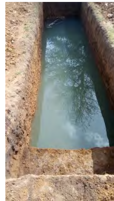
Borehole –Broken, 2 Toilet being excavated filled
