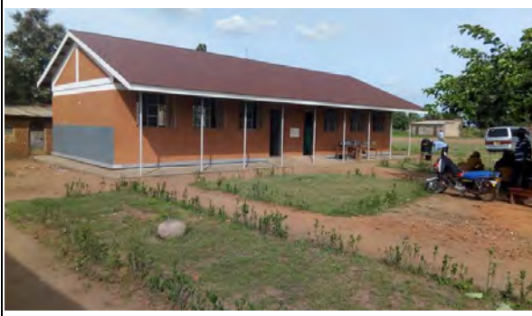
Classroom / Administrative Block -Staffroom under tree
