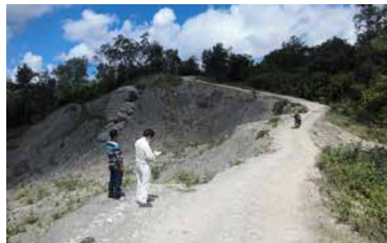
Preliminary survey “Capacity Development for Road Maintenance Maintenance with the Case of National Road No. 1 in Timor Leste”
