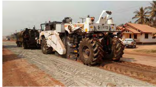
Crushing & mixing by stabilizer
