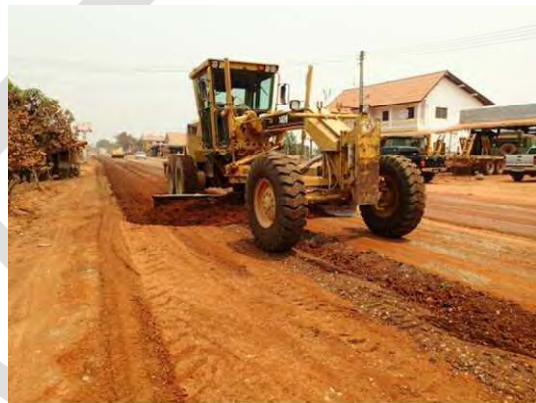
Forming road surface by grader
