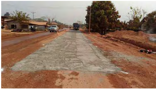
Place cement on existing road surface
