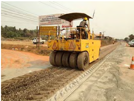
Initial compaction by tire roller
