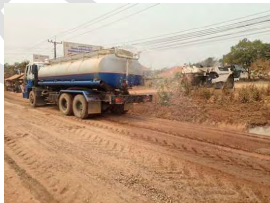
Spraying water on road surface
