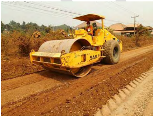
Finishing compaction by steel wheel roller
