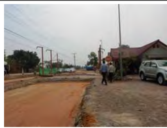
Scarifying existing pavement and sub-grade preparation
