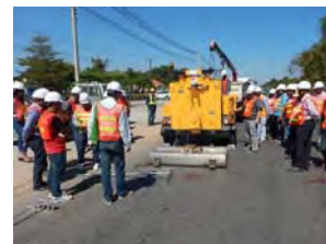
Heating by Road heater
