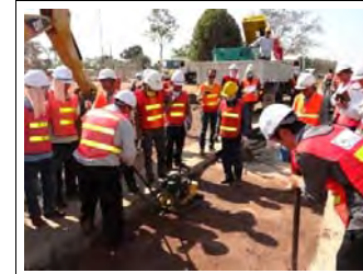
22/Jan: Repair work (spot replacement)
