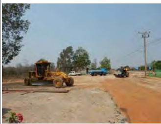
Grading sub-grade
