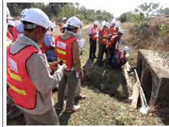
22/Jan: Routine inspection (culvert)
