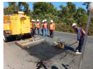
Compaction by Plate Compactor
