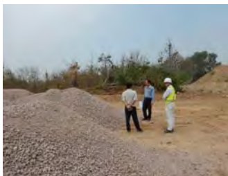
Stockpile of base course material
