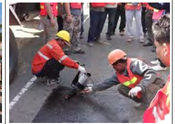
22/Jan: Repair work (crack seal)
