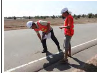
22/Jan: Detailed inspection (pavement)
