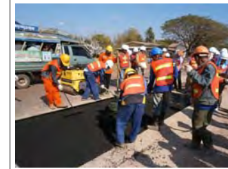
22/Jan: Repair work (spot replacement)
