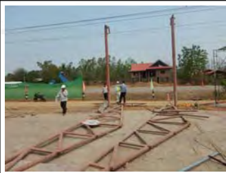
Removing existing roof
