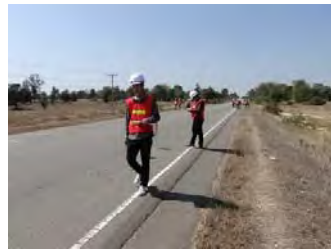
22/Jan: Detailed inspection (pavement)
