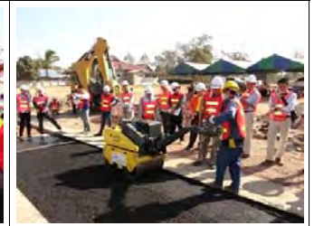
22/Jan: Repair work (spot replacement)
