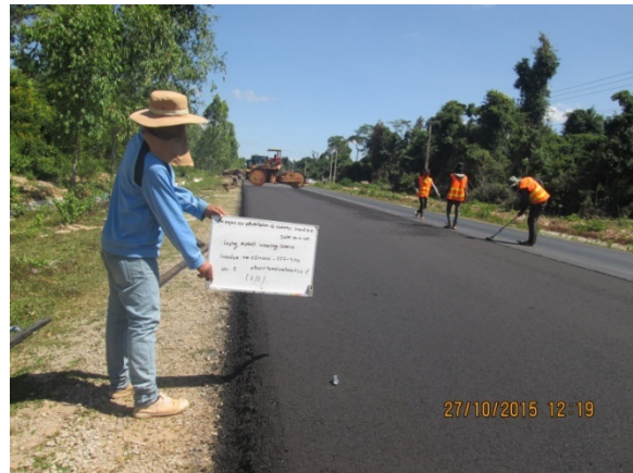
Completion of Compaction
