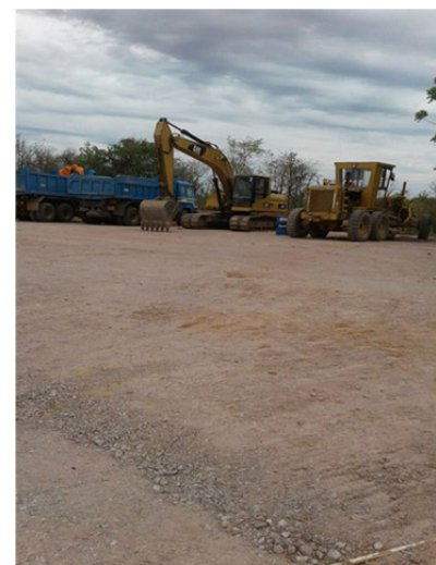
Finishing surface of base course.
