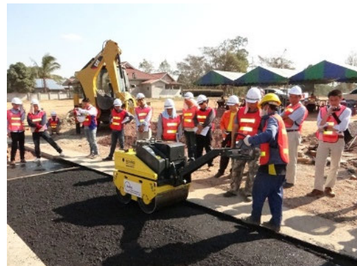
Repair work (spot replacement)
