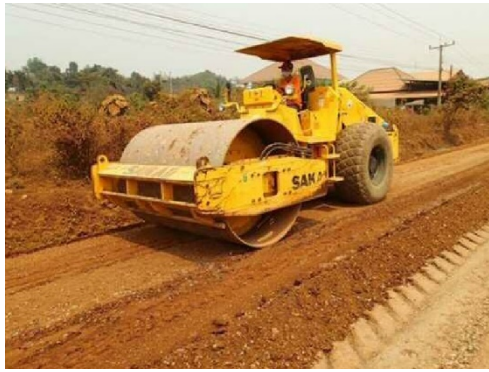
Finishing compaction by steel wheel roller
