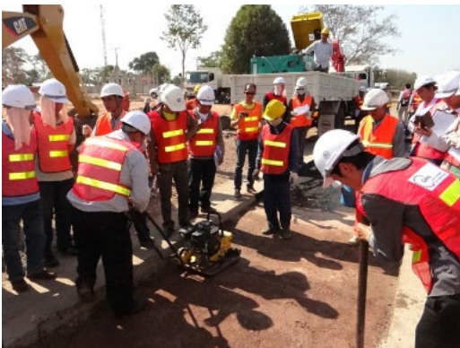
Repair work (spot replacement)
