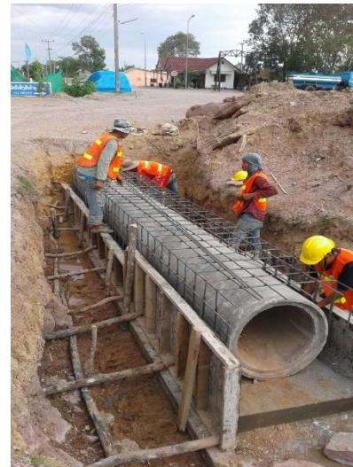
Install pipe culvert.
