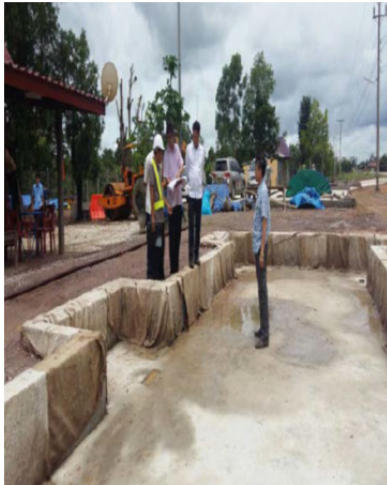
Curing of concrete of the scale foundation.
