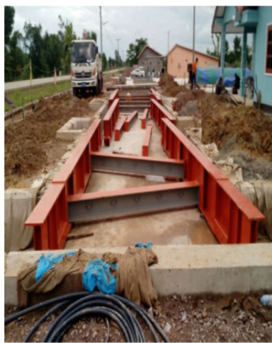
Place steel frame for the platform.
