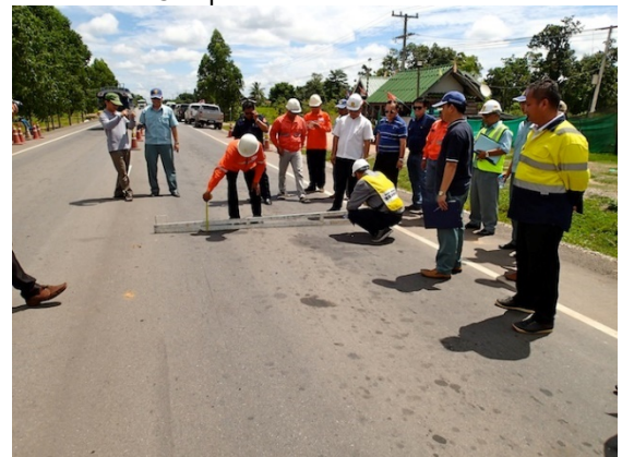
Inspection for Section 3(26th Sep2016)
