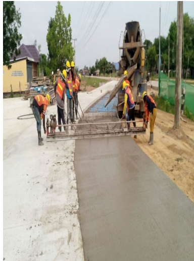
Finishing surface of concrete pavement.
