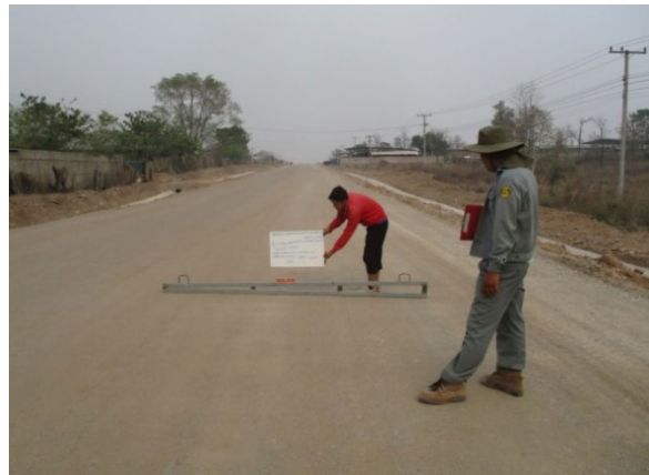
Completion of Base Course work
