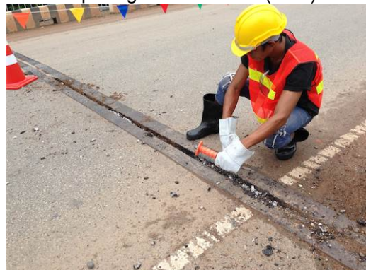
Repairing of Expansion Joint
