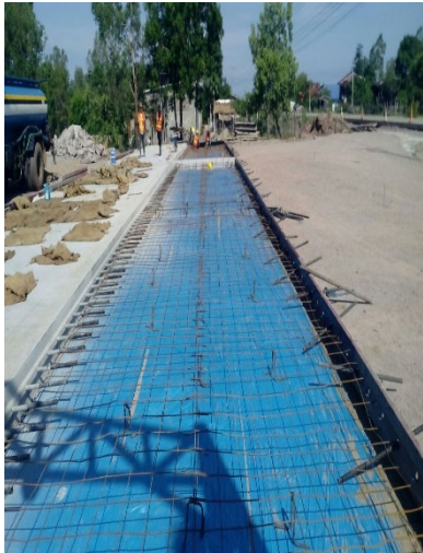
Placing wire-mesh on concrete pavement.
