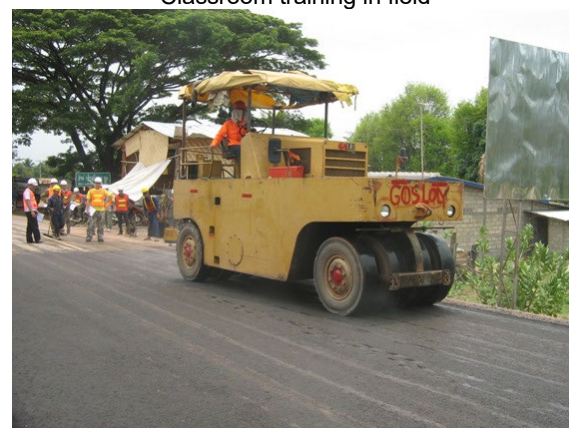
Compaction by tire roller
