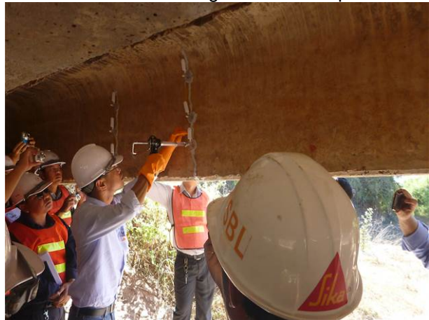
Demonstration of Crack sealing
