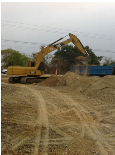
Scarifying existing ground.
