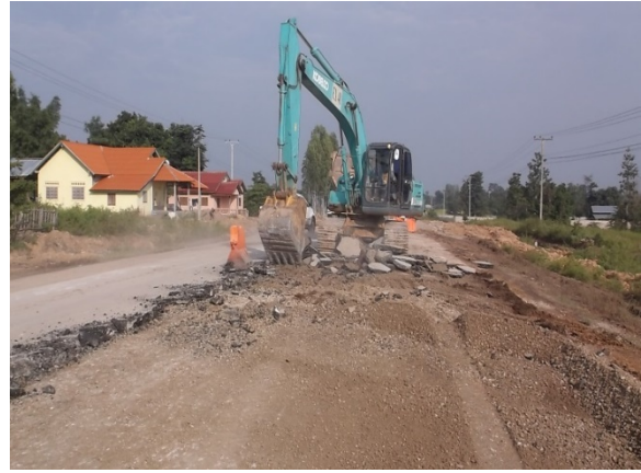
Removal of Existing Asphalt Pavement
