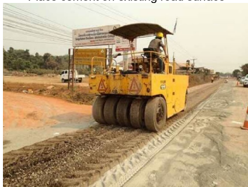
Initial compaction by tire roller
