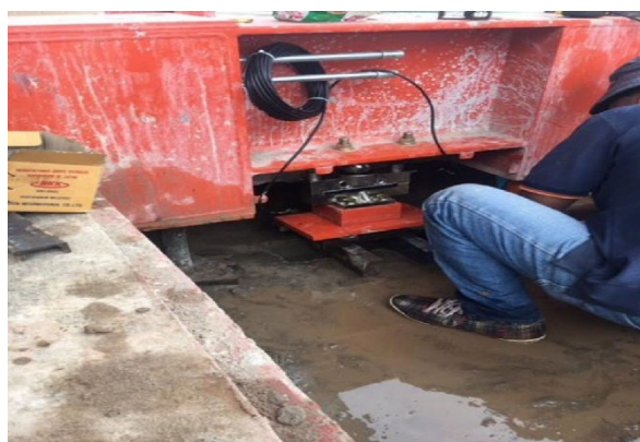
Place load cell for measurement.
