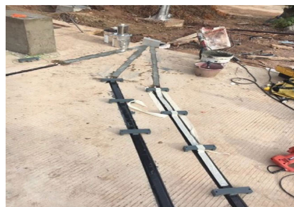
Place sensor of detecting vehicle.
