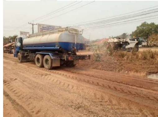
Spraying water on road surface
