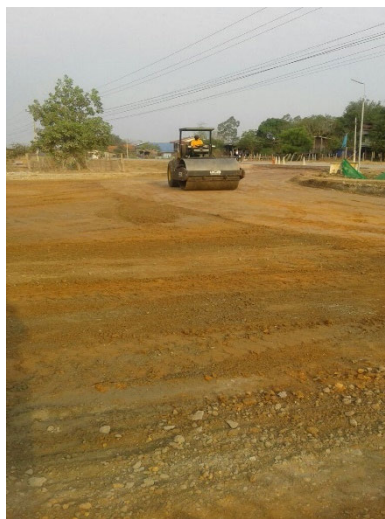
Compaction of sub-grade.
