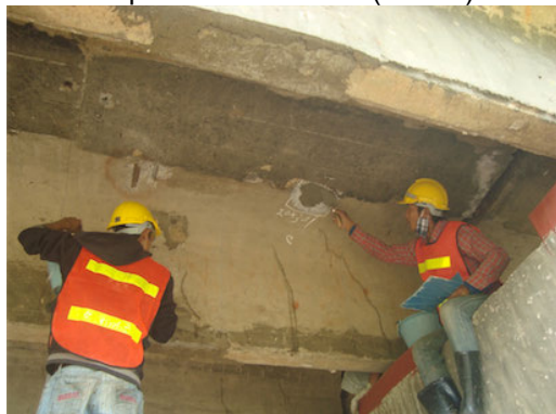
Repairing of Slap
