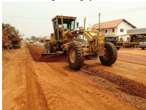
Forming road surface by grader
