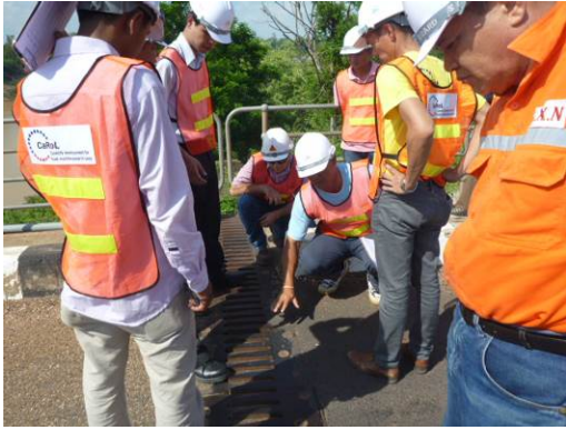
Inspection of Expansion Joint Source: JICA Expert Team
