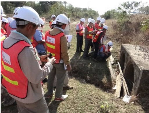
Routine inspection (culvert)
