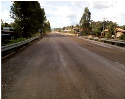
Repair of Base Course
