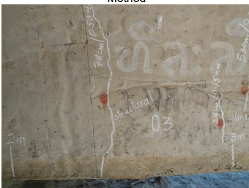
Method of Determine the quantities of Damage
