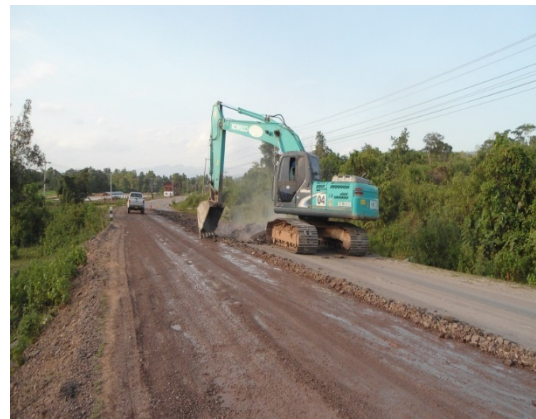
Removal of Existing Asphalt Pavement
