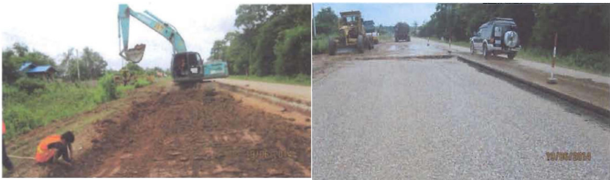
Removal of deteriorated material Source: JICA Expert Team
