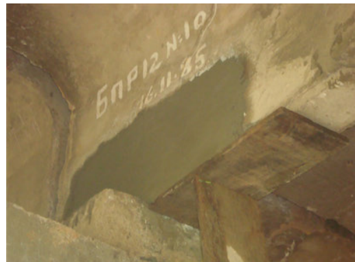
Repairing of Main Girder (After)
