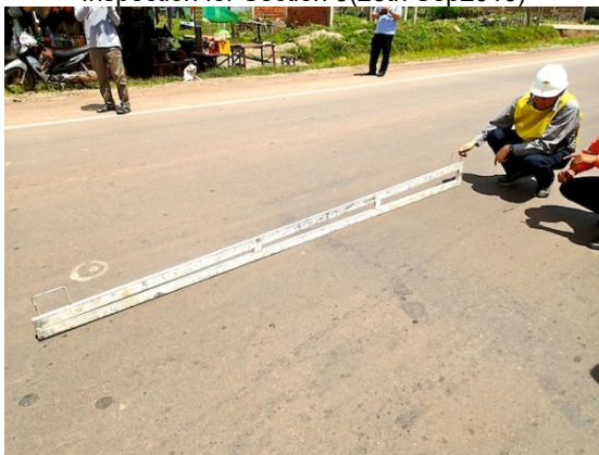
Inspection for Section 3(26th Sep2016)
