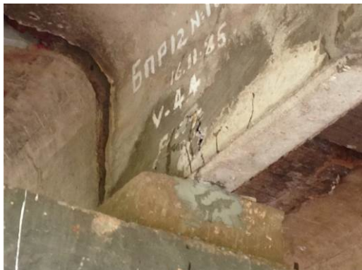
Repair of Main Girder (Before)
