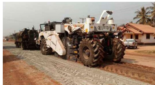
Crushing & mixing by stabilizer
