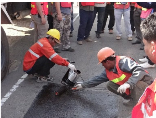
Repair work (crack seal)
