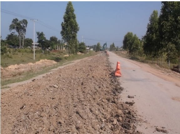
Removal of unsuitable material
