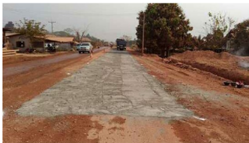
Place cement on existing road surface
