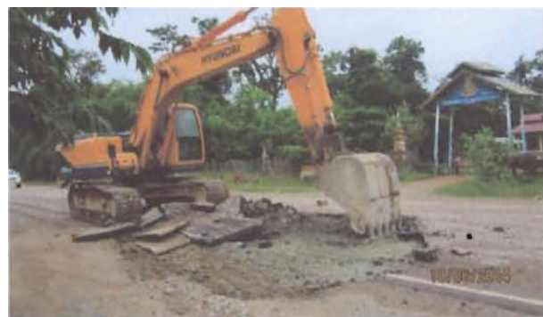
Removal of existing pavement
