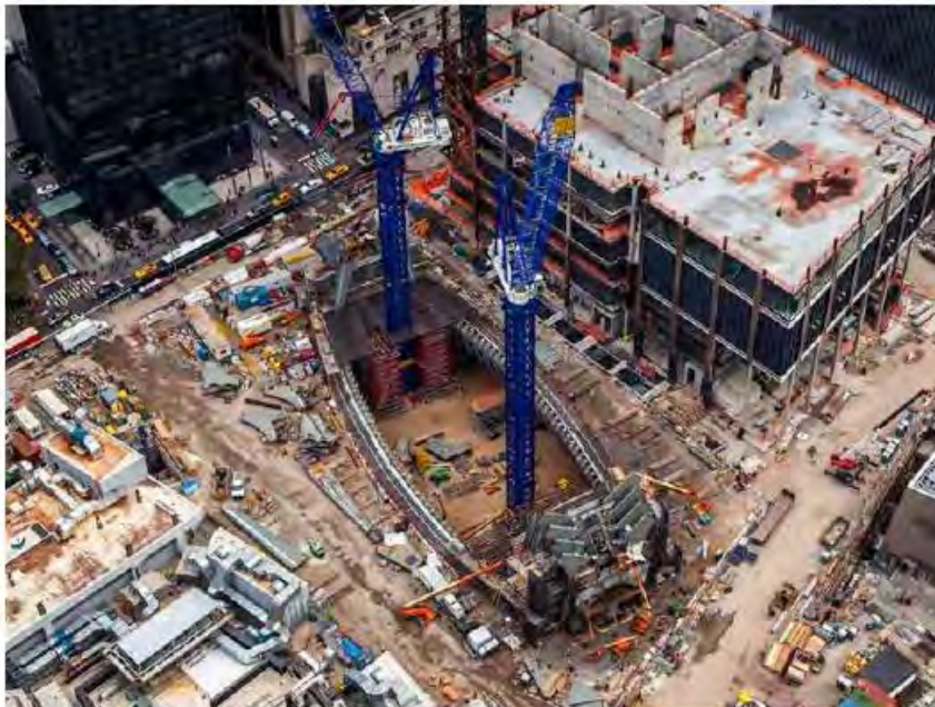
Image credit: Joe Woolhead Courtesy of: Silverstein Properties Taken: September 01, 2013 ※ http://www.wtc.com/media/images/s/wtc-construction-wtc-transportation-hub
