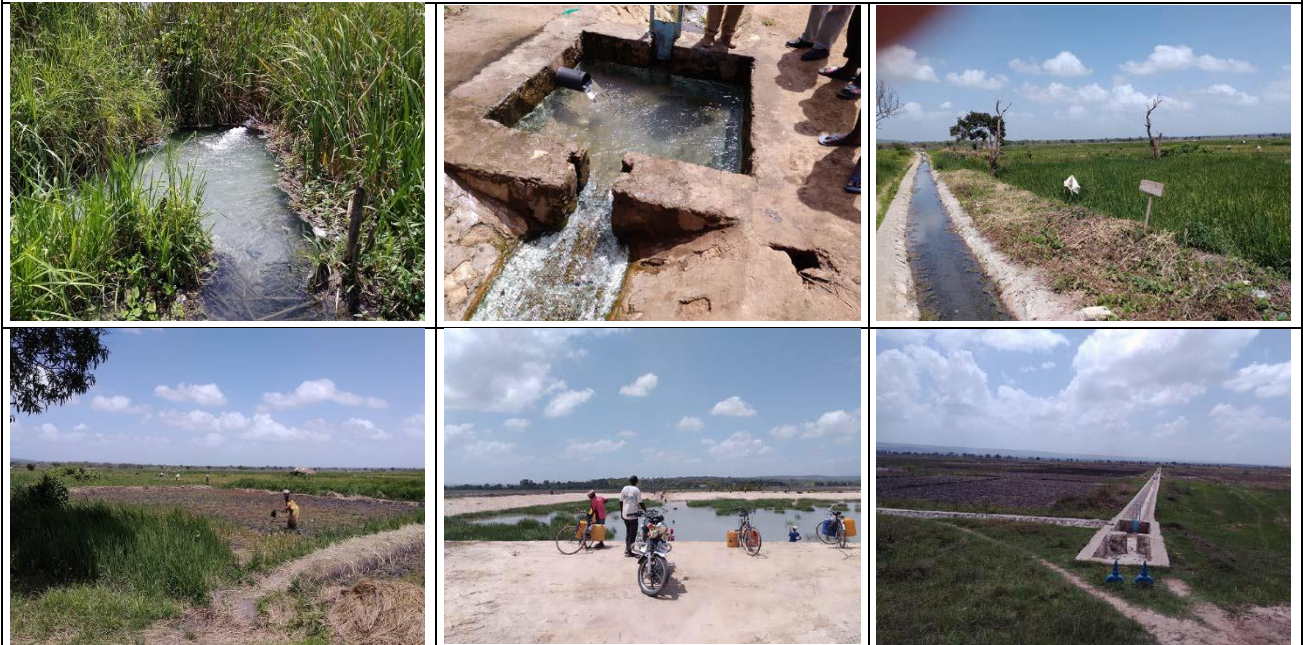
10. Kitere Groundwater Irrigation Scheme, Mtwara District, Mtwara Zone
