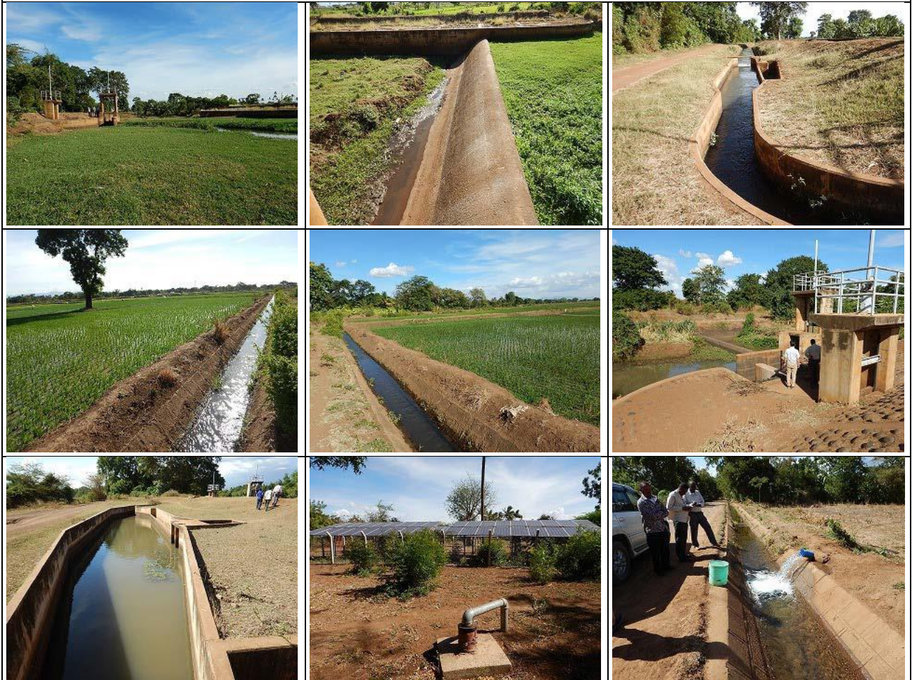
05. Lower Moshi Weir Irrigation Scheme, Moshi District, Kilimanjaro Zone
