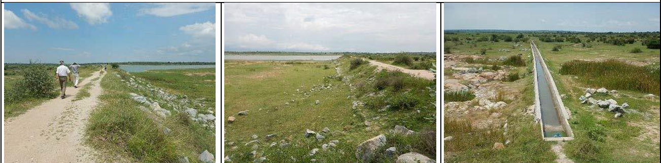
03. Mahiga Dam Irrigation Scheme, Kwimba District, Mwanza Zone
