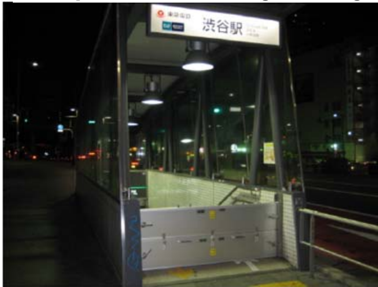
Photo: Examples of water stops installed
