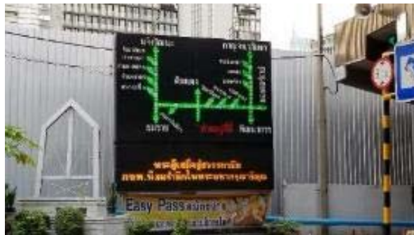
ITS system : VMS at Nana
