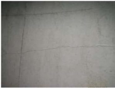
Shrinkage by temperature or moisture
