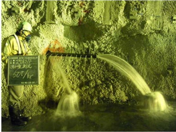
Drainage boring of Kanayama Gero Tunnel
