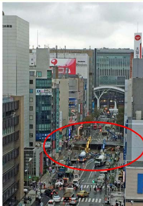
Road subsidence collapse accident in Hakata
