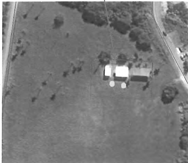
Existing MW mast
