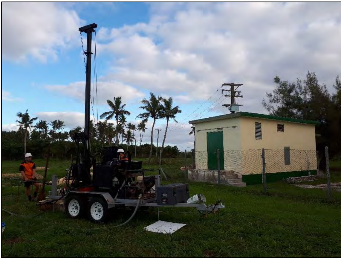
Figure 3.1: Photo of the GDI drill rig used during the investigations, at the TBC MW TX site.
