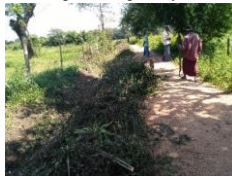
Left bank canal
