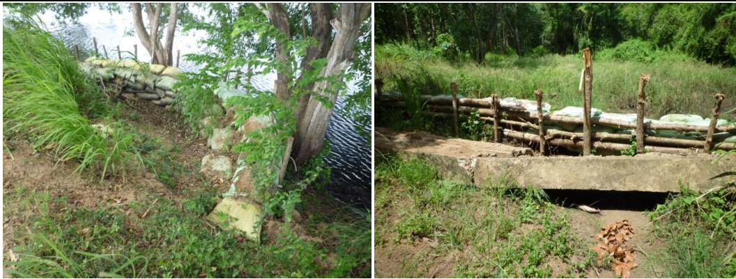
Figure 3.12.7 Examples of Emergency Repair Works (Left: Bund Piping, Right: Spill Collapse)
