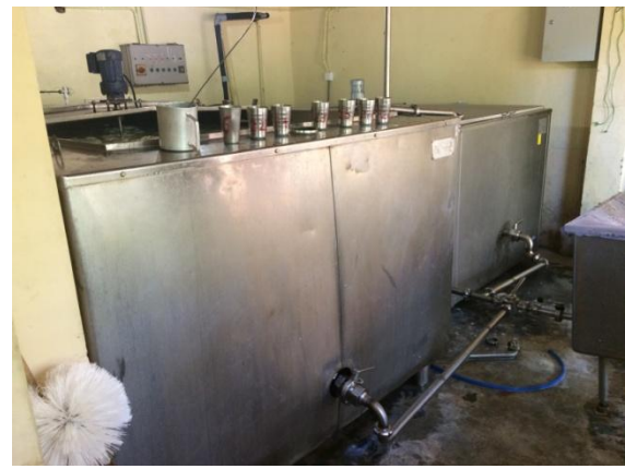
Cooling Facility (Chilling Centre)
