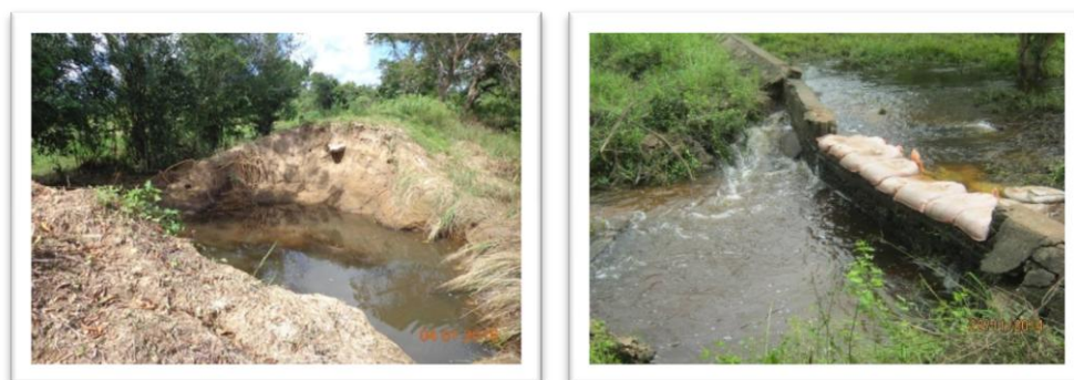
Figure 3.12.5 Tank Disaster due to the 2014 Torrential Rains (Left: tank breach, Right: spill collapse)
