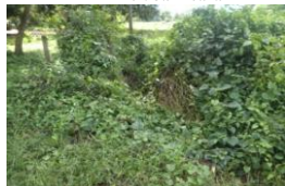
Right bank canal
