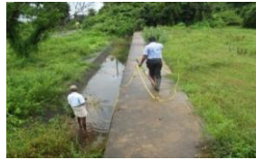
Right bank spillway 1
