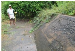
Right bank spillway 2
