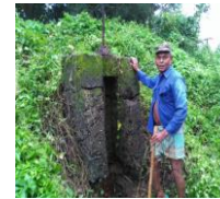
Left bank sluice
