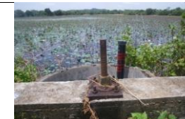
Left bank sluice
