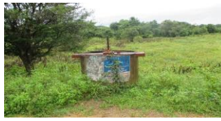
Left bank sluice
