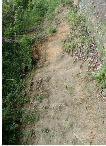
Highly weathered rock on slope
