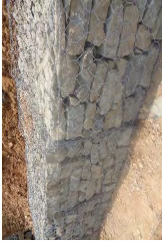
Gabion wall construction in progress
