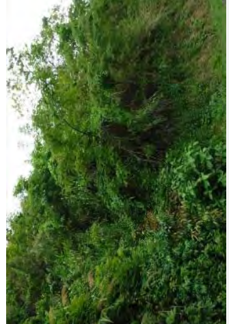
View of slope from the side
