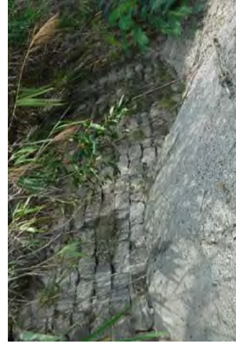
Retaining wall on hill side
