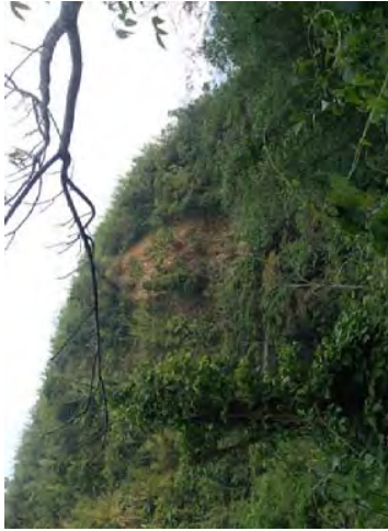
Full view of Critical slope
