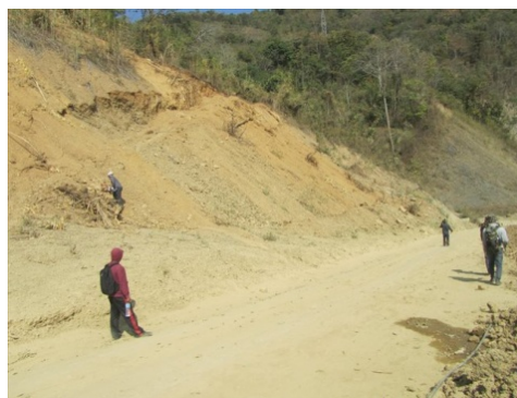
No Deformation on the Road
