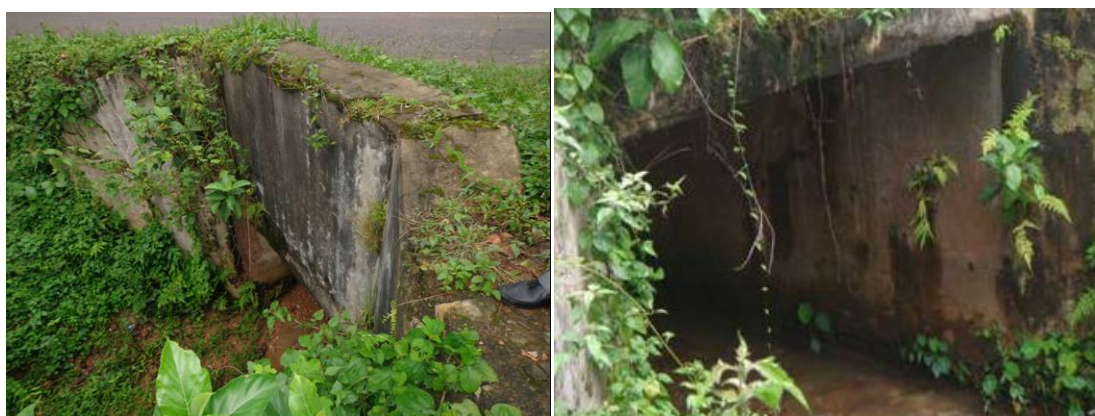
Figure 8.3-8 Example of Existing Slab Culvert
