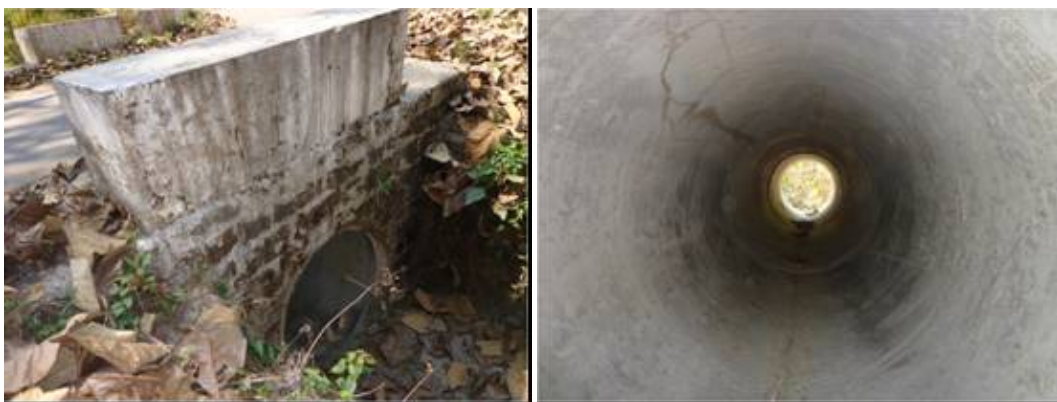
Figure 7.3-21 An Example of Existing RC Hume Pipe
