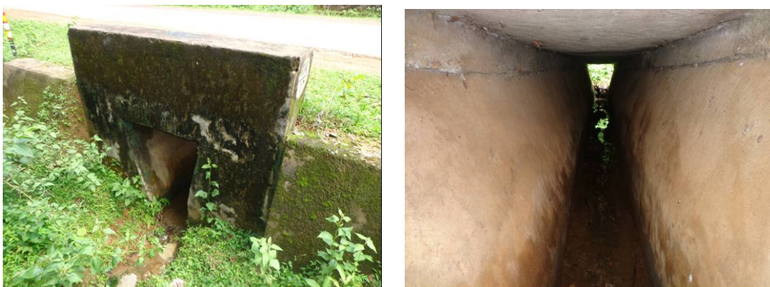
Figure 8.3-9 Example of Existing Slab Culvert with Narrow Inner Width
