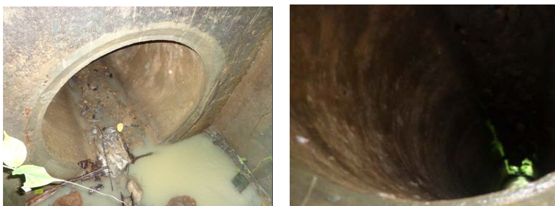
Figure 8.3-10 Example of Existing Pipe Culvert
