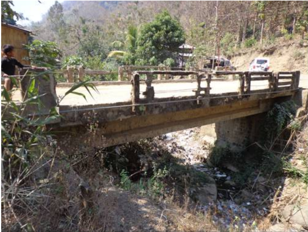
Figure 7.3-4 RC T beam Bridge in Maudarh at 190+190
