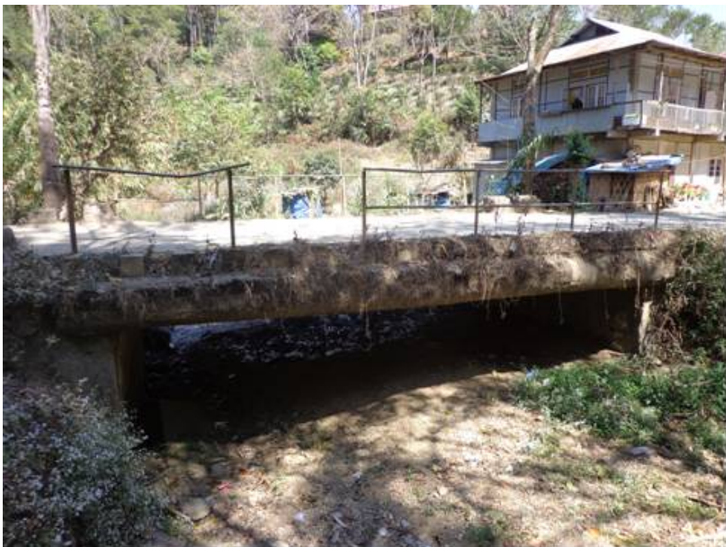
Figure 7.3-5 Slab Bridge in Zobawk at 216+450
