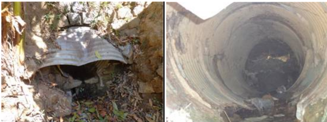
Figure 7.3-22 An Example of Existing GCI Sheet Pipe
