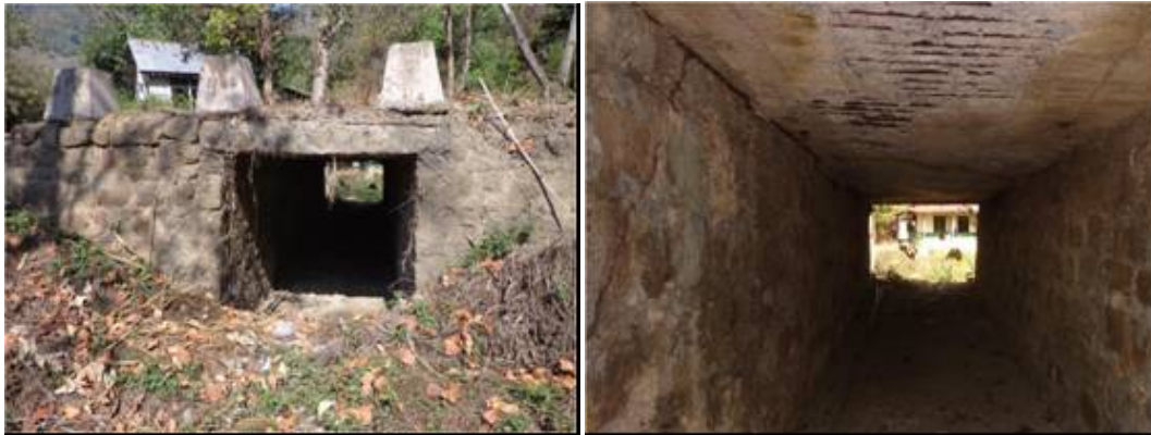
Figure 7.3-20 An Example of Existing Slab Culvert
