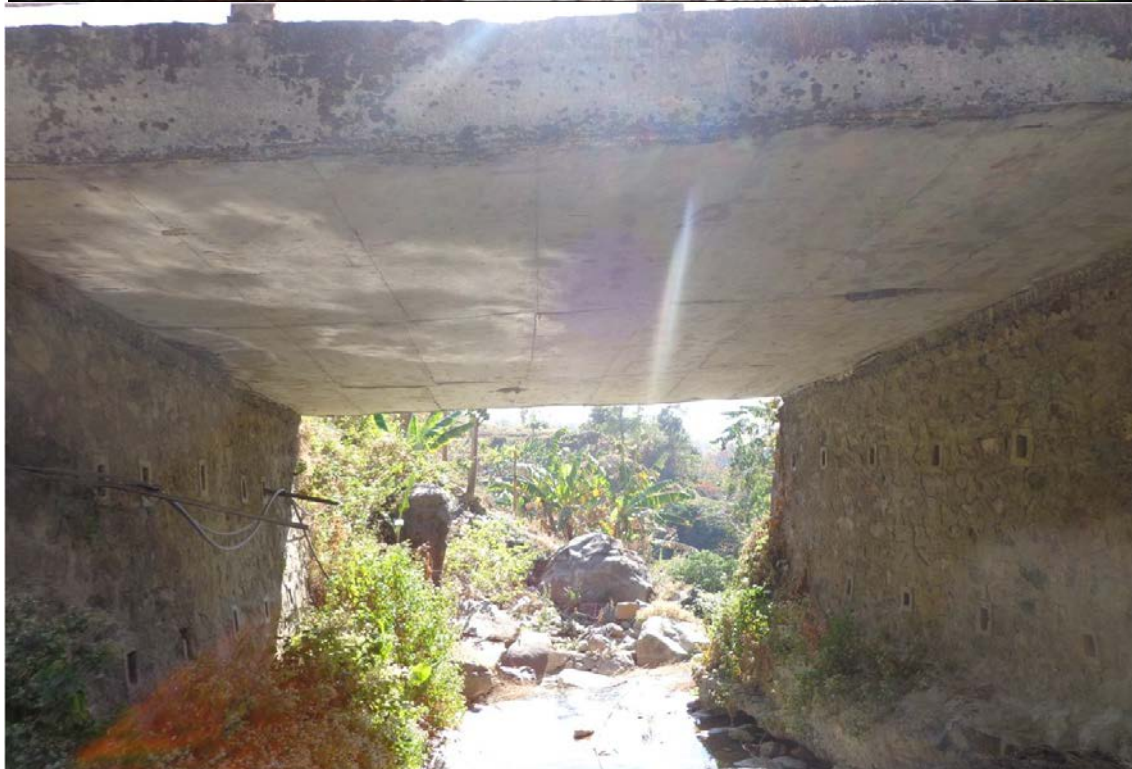
Figure 7.3-23 An Example of Existing Large Slab Culvert
