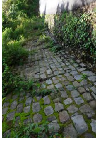
Masonry retaining wall
