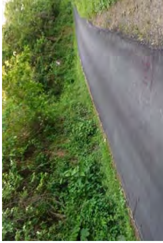
View from beginning point
