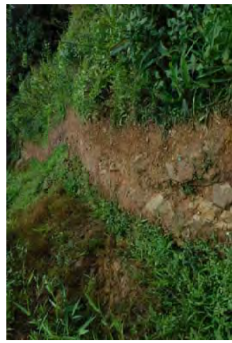
Earthen foot path across lanslide
