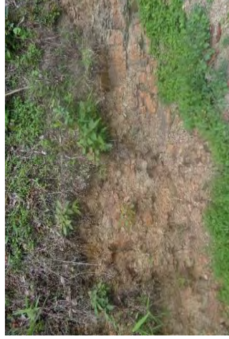
Broken bed rock
