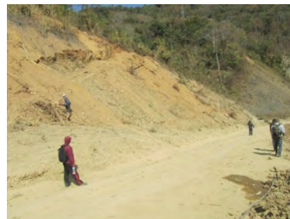
No Deformation on the road
