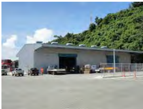
CFS (Container Freight Station)
