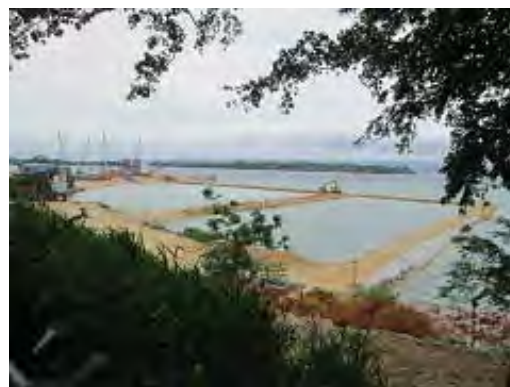
Temporary Storage Area of Dredging Soil
