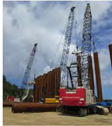
Quay Wall Piling Work
