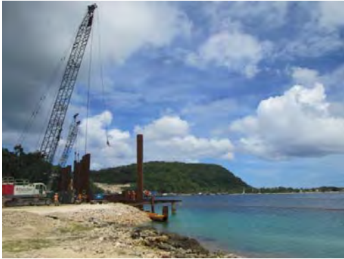
Quay Wall Piling Work
