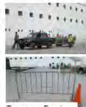
Temporary Fencing (Existing Fence)
