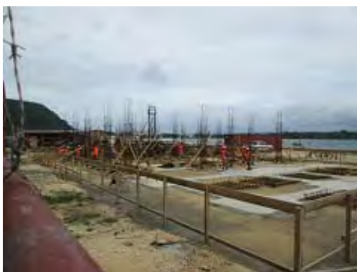
Foundation of Administration Building
