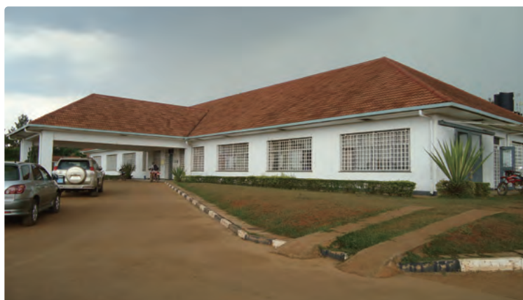
Front View of the Rice Training and Cultivation Centre Building (Research and Administration Block)
