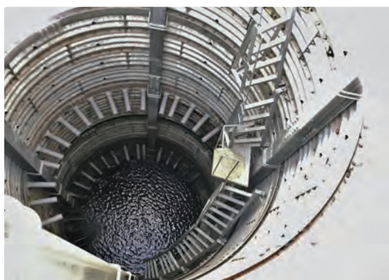
Catchment well and its interior in El Berrinche (water collection boring works deployed in a fan-like fashion can be observed)
