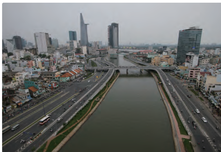
The road constructed under the project on the left (photo provided by construction management consultant)
