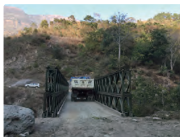
After the construction of Kela Bridge
