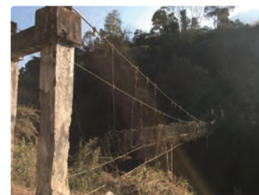
Former Kela Bridge which was a suspension bridge for pedestrians
