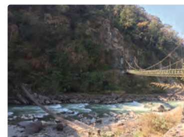
The former (left) and the new (right) Reotala Bridge
