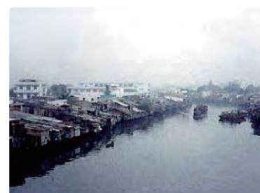
Scenery before the implementation of the project (before rehabilitation of Channel Tàu Hủ Bến Nghé) (photo from the website of Ministry of Foreign Affairs of Japan.)
