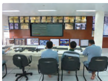
Traffic monitoring by Management Center of Saigon River Tunnel
