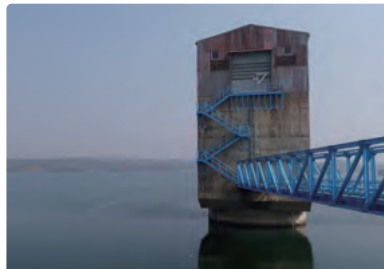
Upper Reservoir and Intake Point
