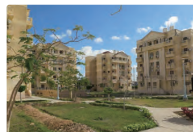
E-JUST Temporary Campus/Dormitories
