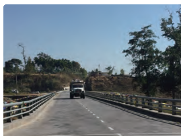
After the construction of Dolkhola Bridge
