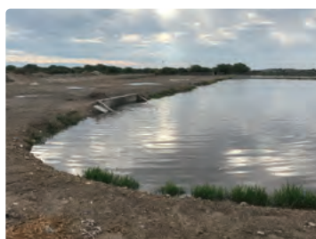
El Indio Sewage Treatment Plant (Piura)
