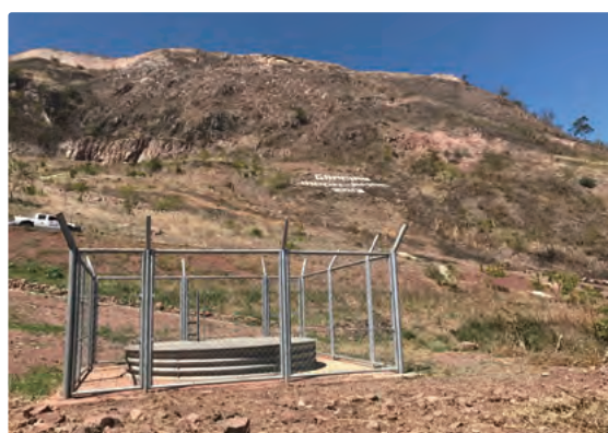
An exterior view of catchment well
