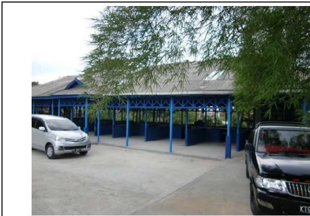
MRF after the Renovation
