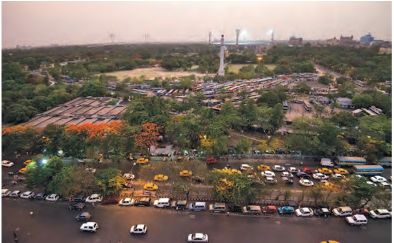
Aerial View of Esplanade showing the Bus Stand (partly) and the Shahid Minar. The Eden Garden Stadium can be spotted in the background of the picture (Photo taken from Grand Hotel).
