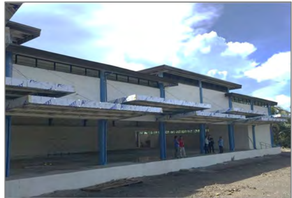
Actual Construction (as of October 2017)
