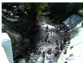
River traversing the Bayabas-Eden Road (Bato Bridge), Toril
