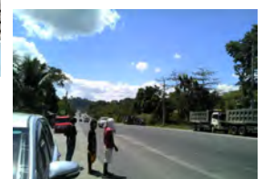
C. P. Garcia (Diversion) Road, Maa Crossing
