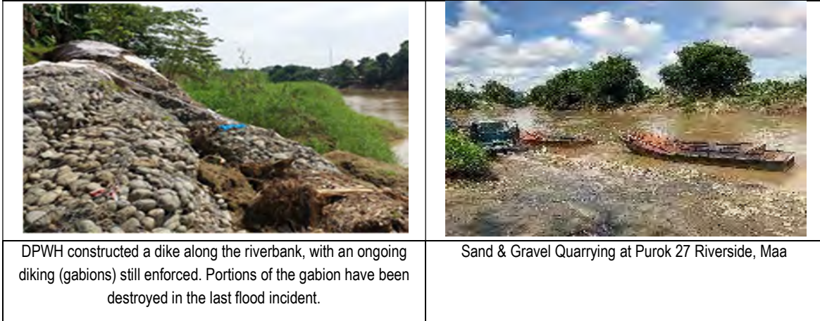
Figure 18.2.6 Destroyed Dike and Sand and Gravel Quarrying
