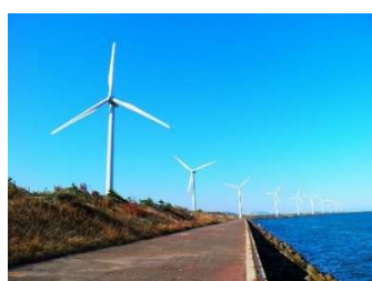
Wind Power Station
