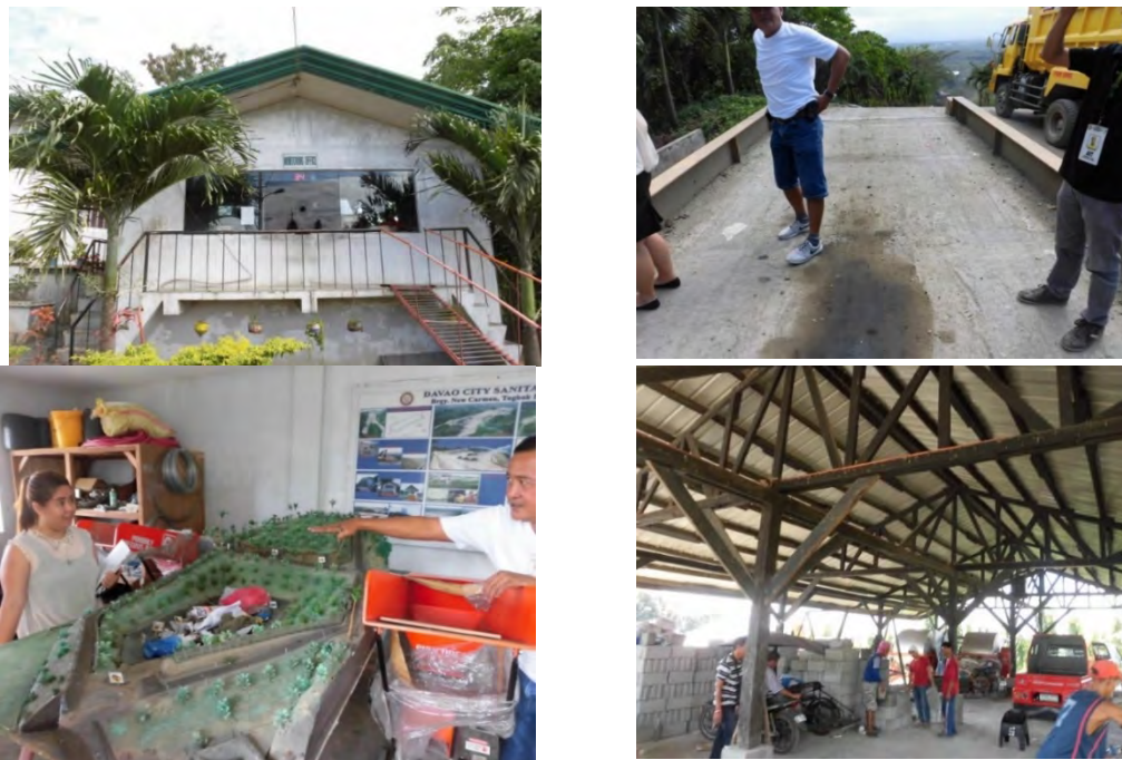
From top left clockwise: weighbridge office, weighbridge body, overall 3D model of the facility, MRF Source: IM4Davao Team
