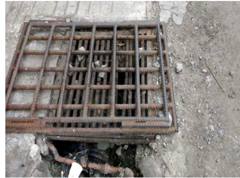
Roadside ditch to storm water pipe
