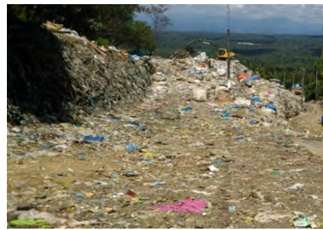
New access road to cell
