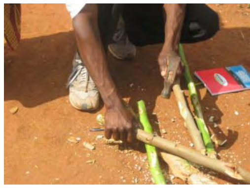
6) Mitengo iwiriyo tiyipingase ndikuyimangirira ndichingwe ndi kukhoma misomali pamene tinayika chizindikiro
