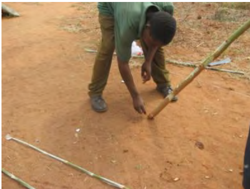
11) Tiyike zizindikiro pamene mitengo yoyimayo inayima ndicholinga choti tikamayigoneka isasinthe.
