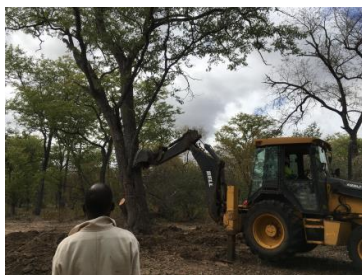
b. Felling the sample tree (by pushing the stem using the arm of an excavator)
