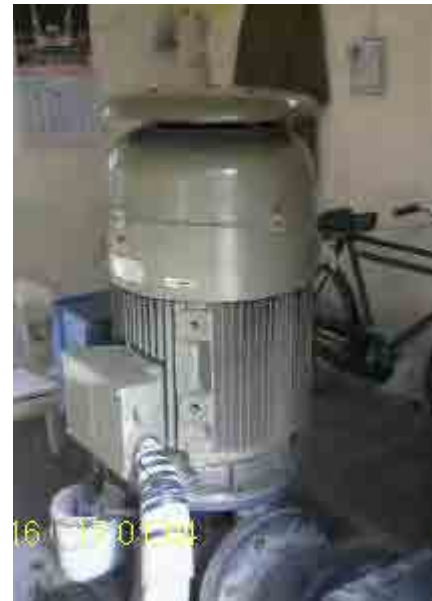
Figure 2 : Excellent Condition of Priming Box and Insulation of cable of Motor Terminal Box
