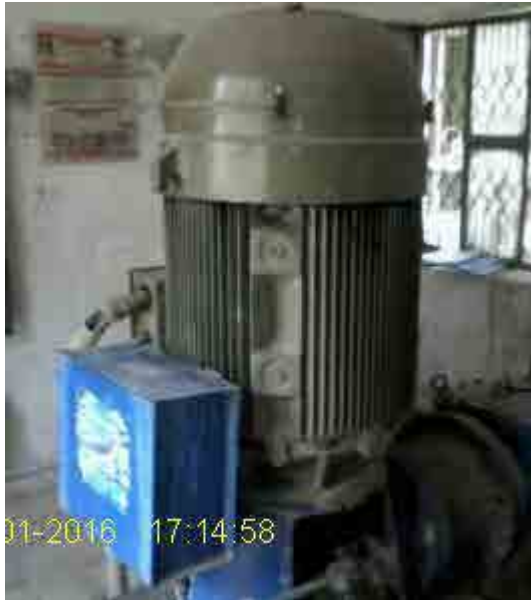
Figure 2 : Excellent Condition of Priming Box and Insulation of cable of Motor Terminal Box
