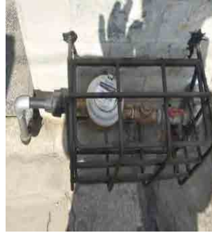
Correct Installation (Horizontally)
