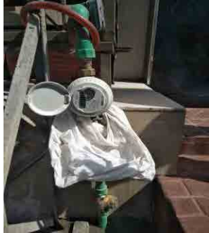
Wrong Installation (Vertically)
