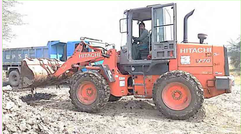
Accident due to vision obstruction / frequent movement
