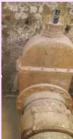
Corrosion and Contamination
