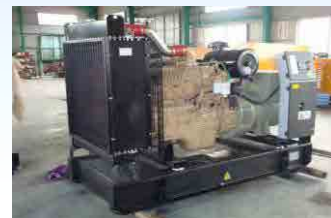
Main frame of Diesel Generator
