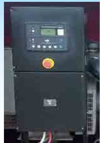
Electrical Control panel
