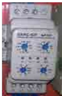
Under/Over Voltage Relay
