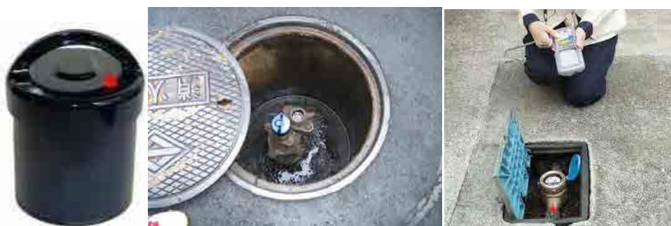
Figure 14: L-sign Install at a fire hydrant (Source: Suido-tec. Co., Ltd.)
