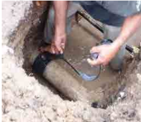
Figure 13: Joint with Rubber Tube
