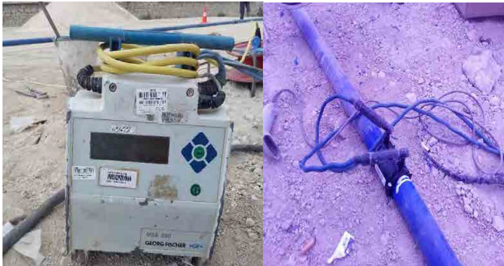
Figure 22: Electrofusion Fitting
