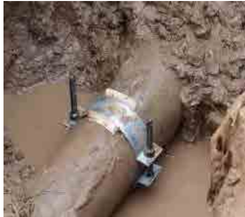
Figure 11: Clamp Joint
