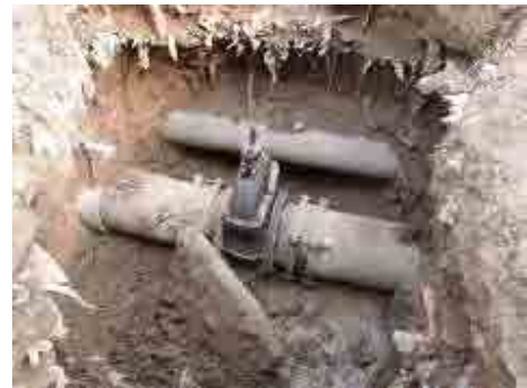
Figure 9: Gibault Joint
