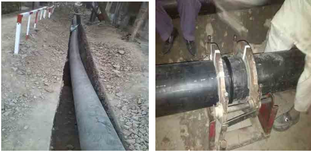
Figure 20: Molded Butt Fusion
