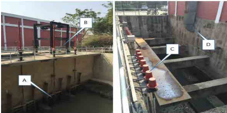
Water level censer, Penstock valve, Exhaust duct, Screen facility
