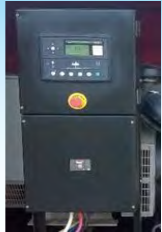
Electrical Control panel
