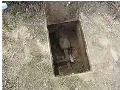
Meter almost buried in the soil
