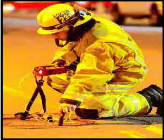
Gas Monitoring at Manhole
