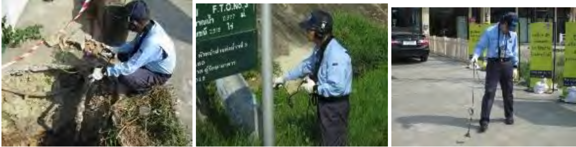
Figure 6: Acoustic Survey with Leak Detector
