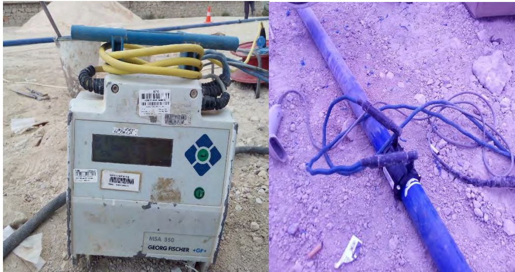
Figure 22: Electrofusion Fitting
