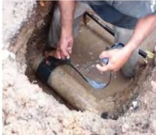
Figure 13: Joint with Rubber Tube
