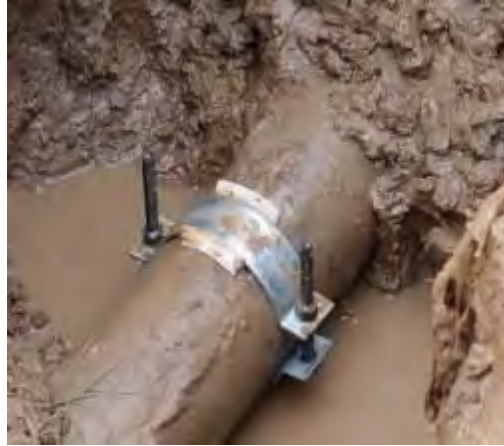
Figure 11: Clamp Joint
