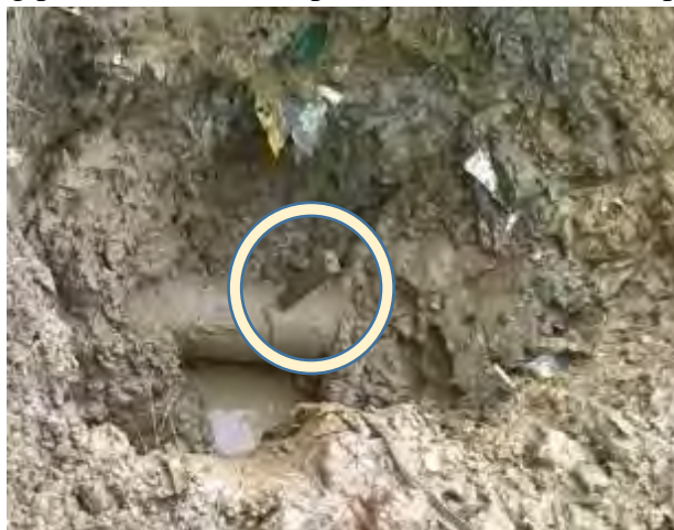
Figure 15: Cork Joint
