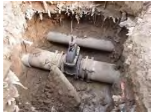
Figure 9: Gibault Joint
