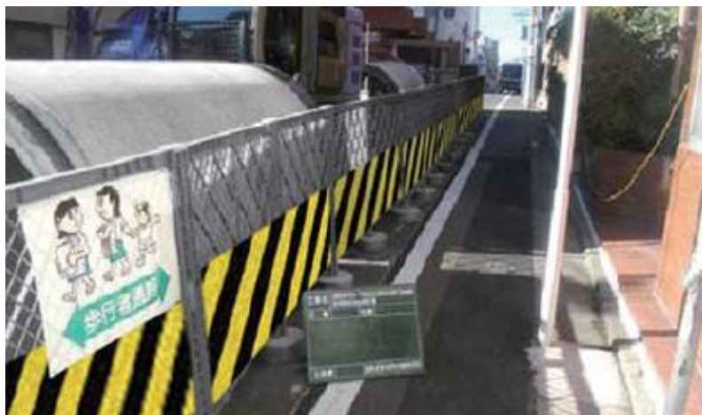
Plate 3: Example of safety sign during construction of water supply system
