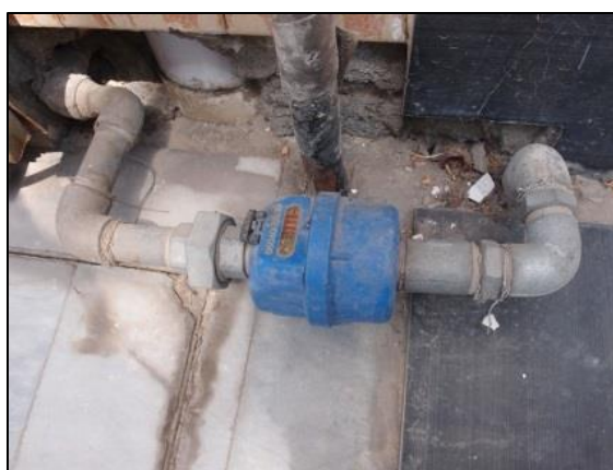
Plate 1: Domestic Meter at Consumer End
