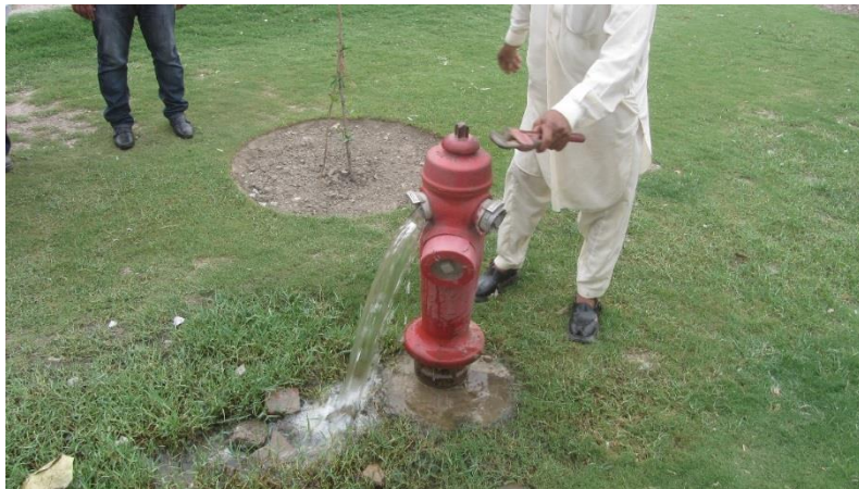
Plate 3: Post Type Fire Hydrant at Green Town, Lahore
