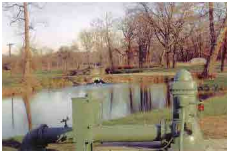
Figure 29 High-capacity turbine pump installed on a municipal well at Rohrsers Island. Recharge lagoon in background
