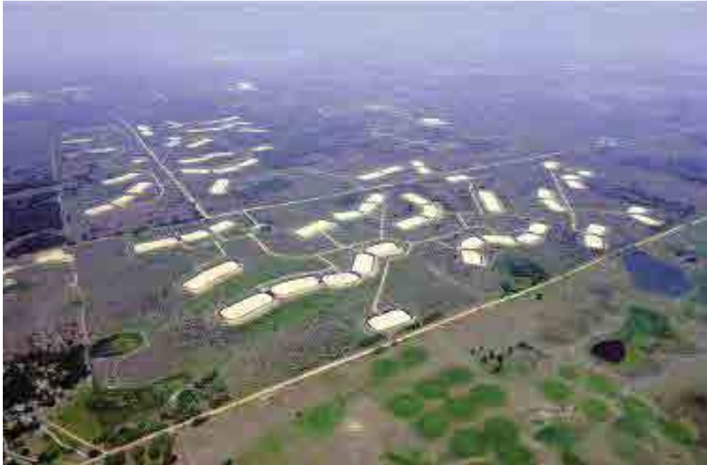
Figure 30 Rapid infiltration basins of Water Conserv II facility, Orlando, Florida
