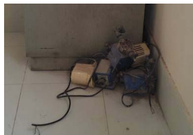
Picture 6.5 Collected Malfunctioned Chlorinators
