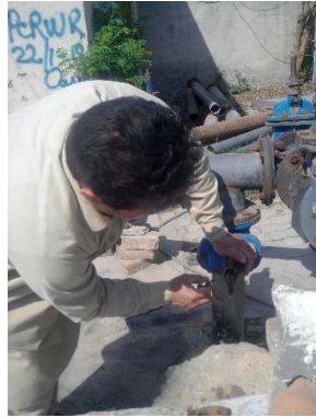
replacement of gland packing
