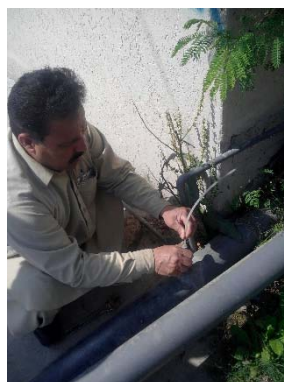
Picture 6.13 Cleaning of Scales Attached in Discharge Nozzle of Chlorinator at Tube Well in East Zone 60B Motimahal
