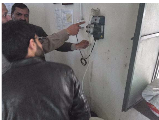
Picture 4.5 Checking chlorine dosage equipment
