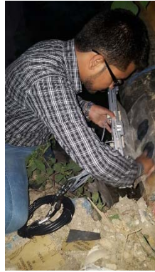
Picture 6.9 Installation and Measurement of Flowrate by Ultrasonic Flow Meter on June 8, 2017
