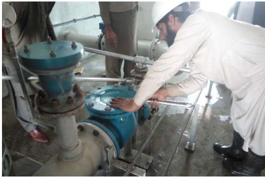
Photo 17: Opening of non-return valve
