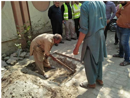
Reaching buried manhole cover
