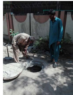
Setting of manhole cover on ground level
