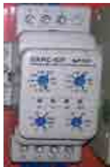
Under/Over Voltage Relay
