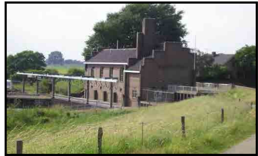
Pumping station - Netherlands
