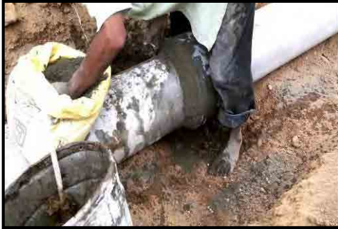
Sewer Pipe Joining Works
