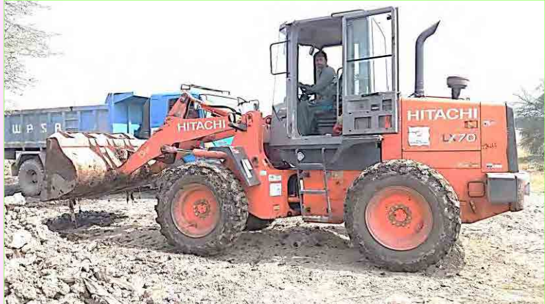
Accident due to vision obstruction / frequent movement
