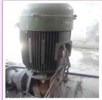
Broken Casing
