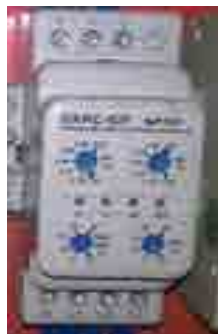
Under/Over Voltage Relay
