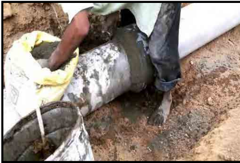
Sewer Pipe Joining Works
