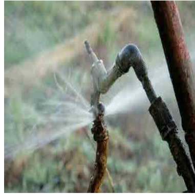
Leakages from meter connections
