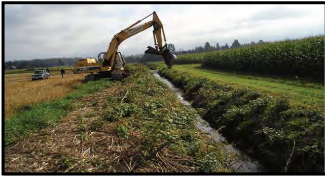
Figure 8: Lidded Bucket on tracked Excavator
