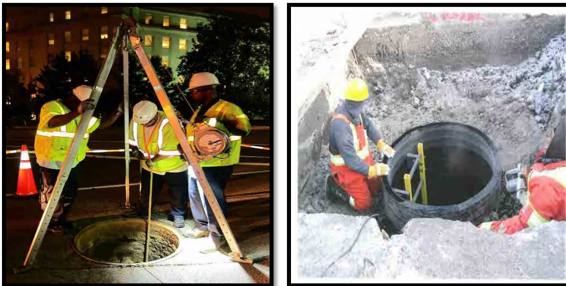
Figure 4: Use of Tripod Stand and Proper Ladder for Manhole Entry
