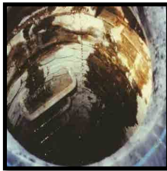
Figure 5 Leaky manhole
