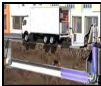
Figure 5: Spirally wound pipe
