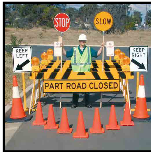
Figure 7: Barricading and Usage of Safety Signs for Traffic Control
