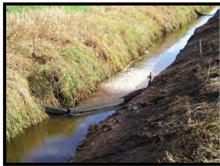
Figure 7: Temporary Silt Fence
