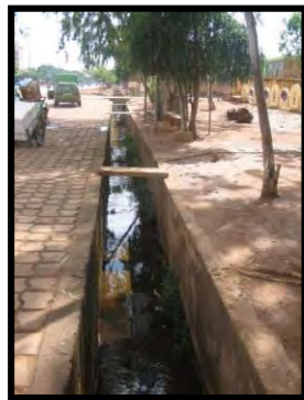
Figure 6: Road-side Open Drain
