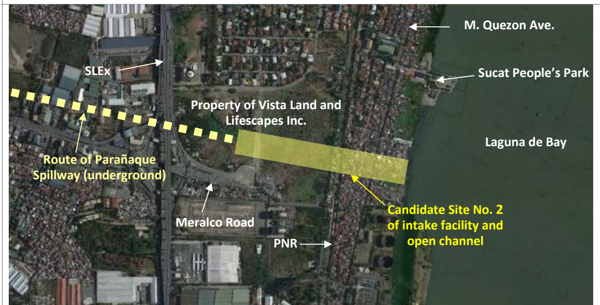
Aero Photo 2 : Candidate Site No. 2 of Intake Facility and Open Channel (Barangay Sucat, Muntinlupa)
