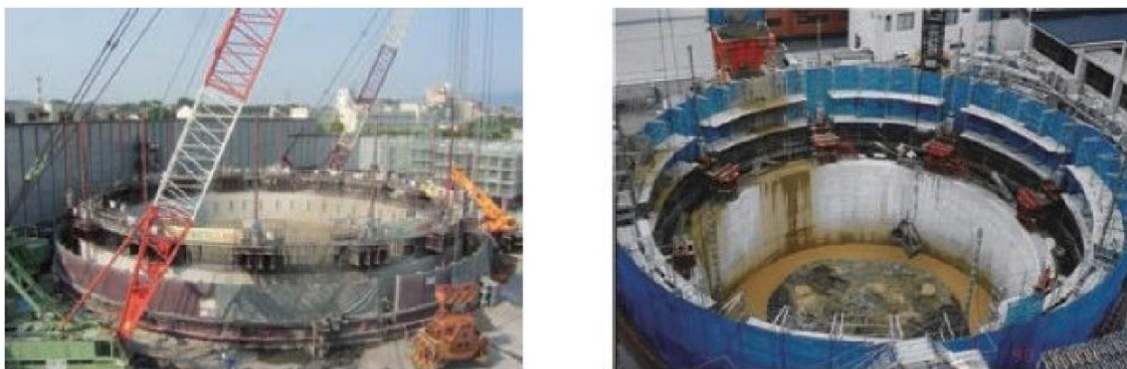
Figure 7.5.13 Photo of Press Caisson Construction
