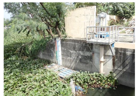
Figure 7.2.24 Water Hyacinth at Suction Side of Pumping Station
