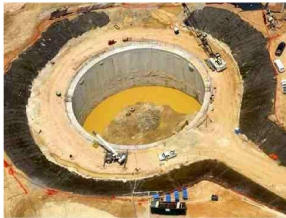
Figure 7.5.10 Case of RC Diaphragm Wall Circular Shaft
