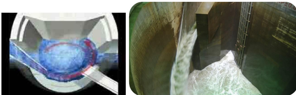
a) Explanation of Vortex Drop Shaft; b) Inflow Situation of August 2005 Flooding (No. 3 Vertical Shaft) Source: http://www.ktr.mlit.go.jp/edogawa/gaikaku/intro/02shuyou/shu-05.html and “Sairyu no Kawa, Metropolitan Area Outer Underground Discharge Channel”
