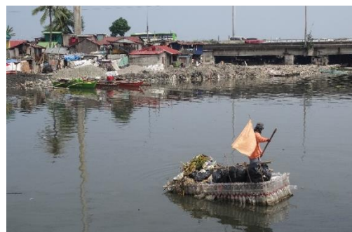
Zapote River Left Bank near Outfall
