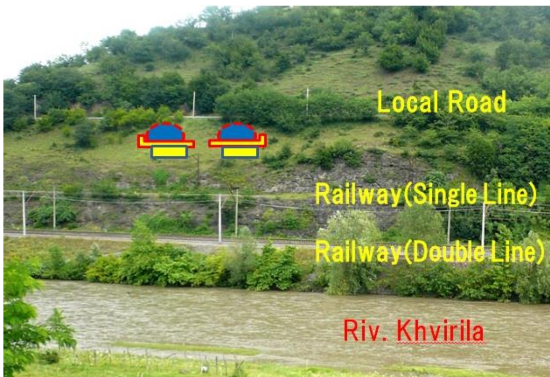
Figure 5-1: Elevation Differences with Related Facilities about BR4004
